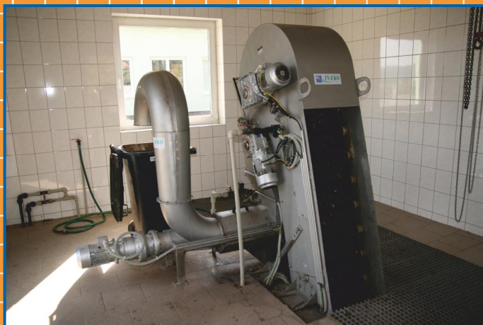
Belt screen and press for screenings
